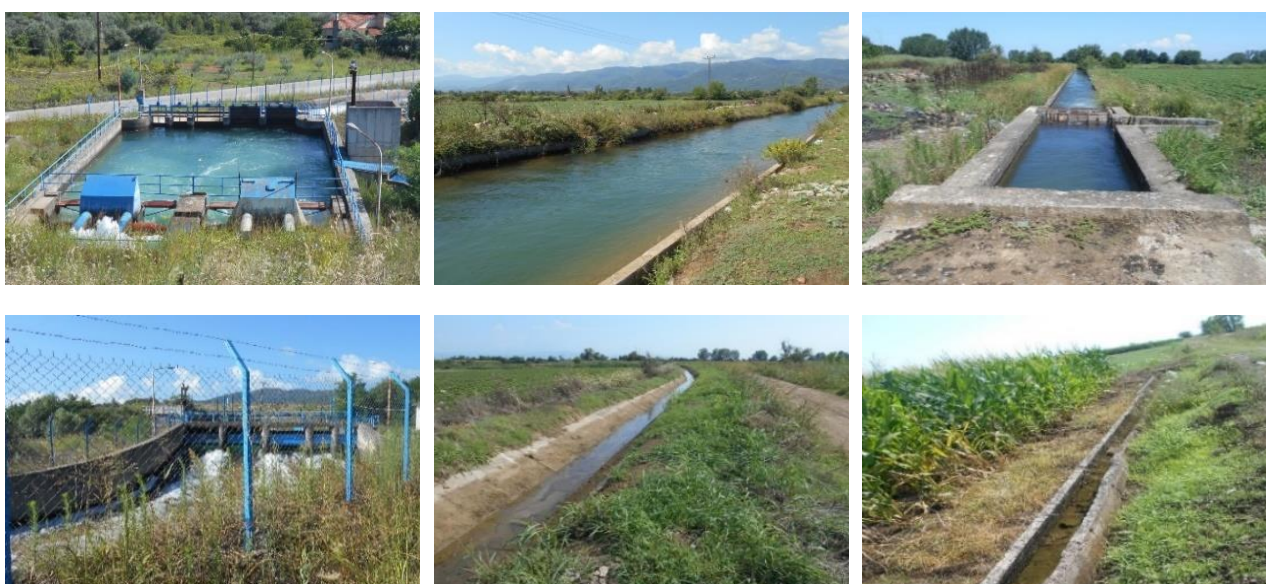
Figures 3-8. Aspects of the existing Land Improvement Infrastructure of Tavropos (irrigation network): water tank, central channel, primary, secondary and tertiary channels
