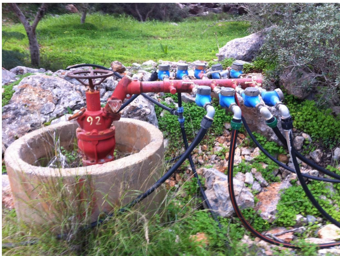
Photo 1. A water uptake serving 9 hydrants in Crete (by A. Stefopoulou)
